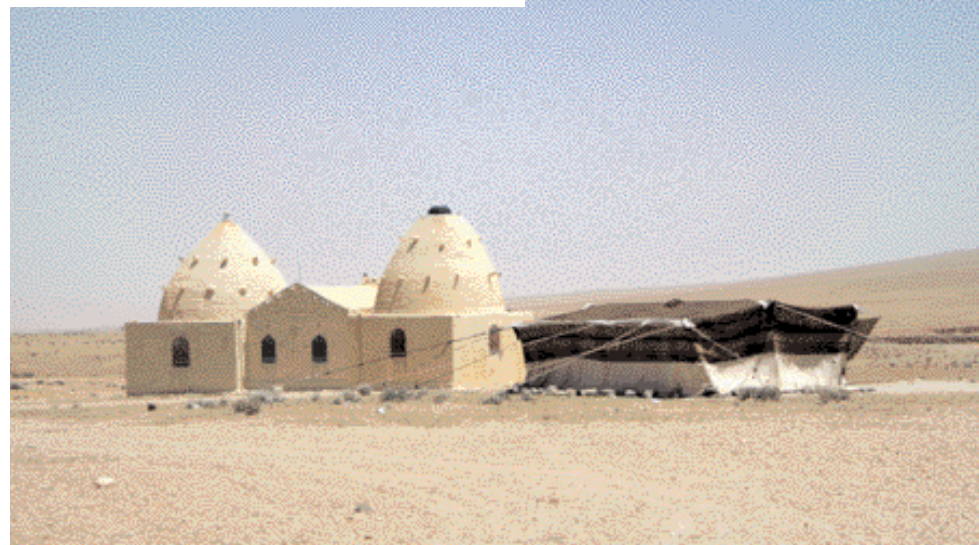
A Syrian Beehive house out of clay, a "Qubab" house, beside a Bedouin tent made of goat hair. Beehive houses are part of the ecological architecture of Syria's country population, their tradition said to be thousands of years old. In a region lacking trees and therefore roof construction material, dome-shaped roofs were
